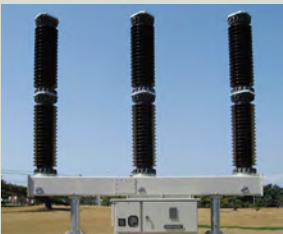
Live Tank circuit breaker
