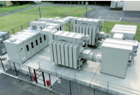
A high-voltage substation for GX at Meidensha's Numazu Works
