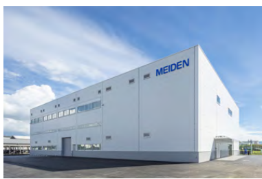
Technical training center (Manabi-ya) (opened in October 2020)
