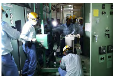
Replacement of equipment
