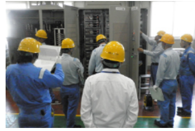
Technology training (high voltage inverter)
