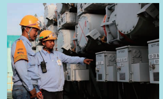
150 kV gas-insulated switchgear on-site testing
