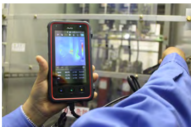
Thermal imaging analysis at walk through
