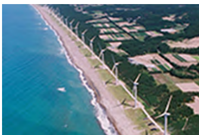
Hachiryu Wind Farm
