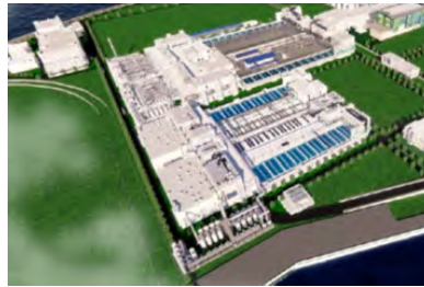
Tuas Water Reclamation Plant
