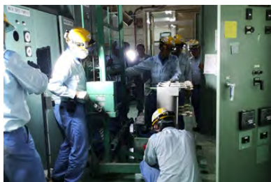
Replacement of equipment
