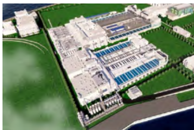
Tuas Water Reclamation Plant
