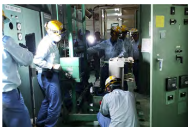
Replacement of equipment
