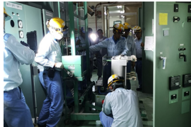
Replacement of equipment
