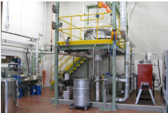
Dissolution plant exterior
