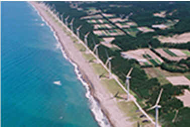
Hachiryu Wind Farm
