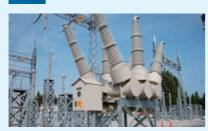
Electricity generated at each power station goes through transmission lines, substations, and distribution lines. As it goes, the voltage is adjusted at each stage before being delivered to factories, buildings and our homes. Meiden transformers change (transform) voltage, while Meiden breakers cut off the large amounts of current that occur in accidents. These Meiden products are essential for safe and reliable electricity transmission and distribution.
