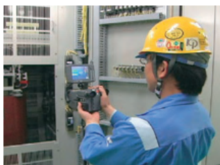
Facility diagnosis at the power "on" condition
