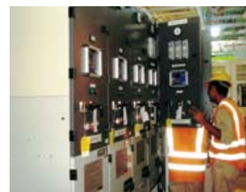
Direct current breaker for railway use
