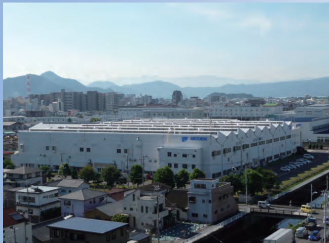
▲ External view of Component Factory
