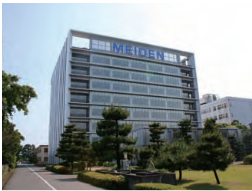
The main building of Meiden Numazu Works
