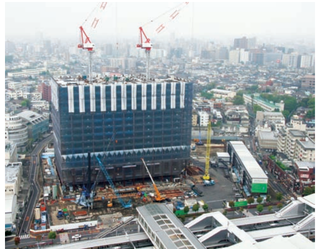
Construction site (as of April 2006)
