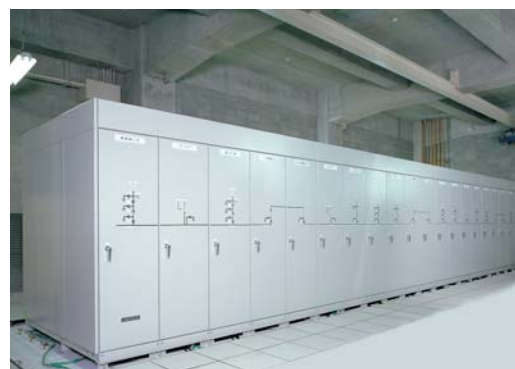
36kV cubicle-type gas-insulated switchgear (C-GIS)
