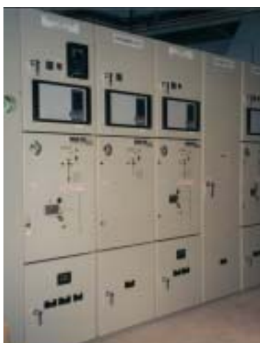
22kV gas-insulated switchgear for traction substation
