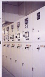
12kV Metal-clad Switchgear, HICLAD-10J
